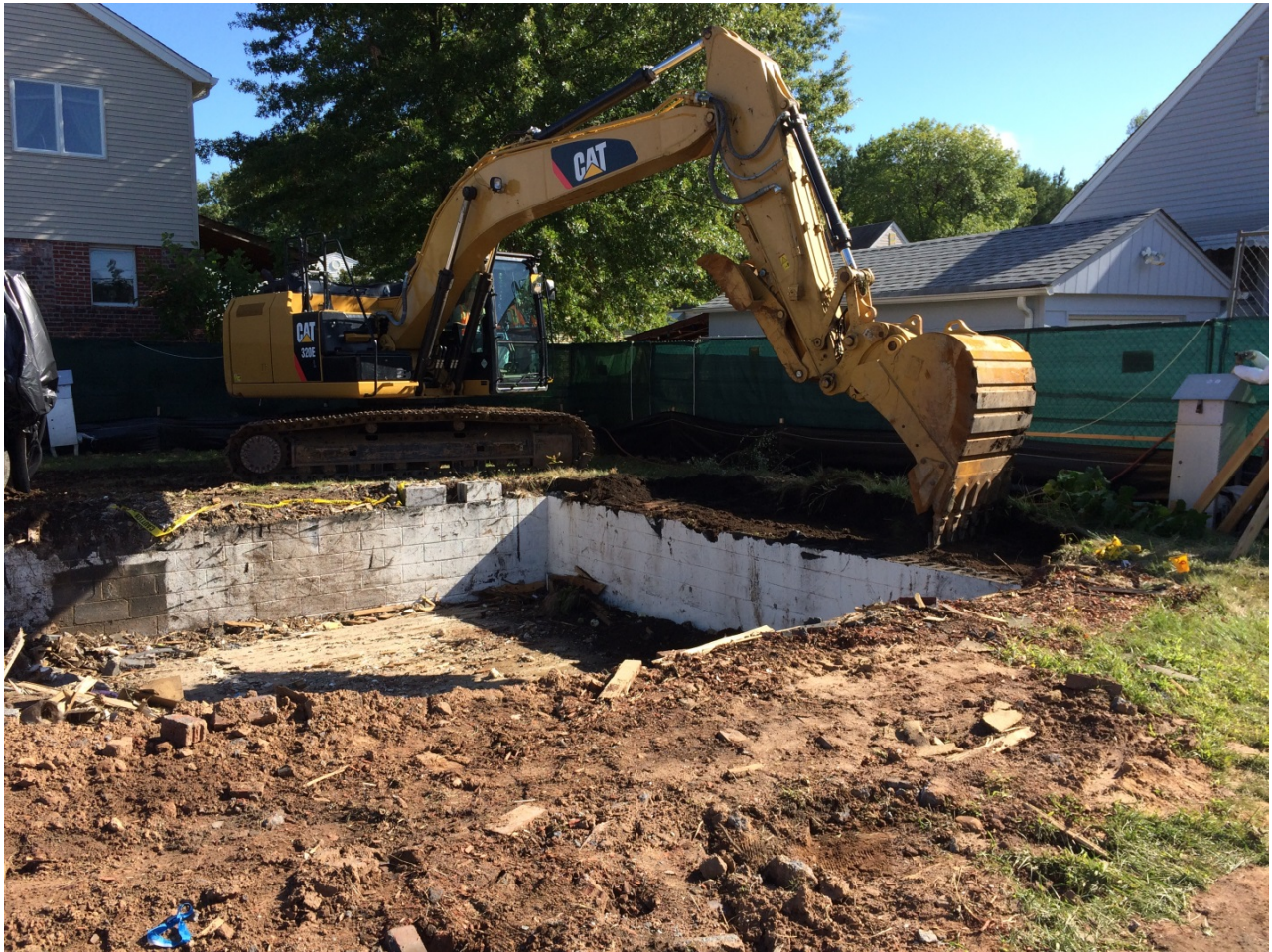
Fig. 3. 61 Trudy Drive during demolition. Note the proximity of the neighboring homes (4 Hancock Street on left, 63 Trudy Drive on right).
