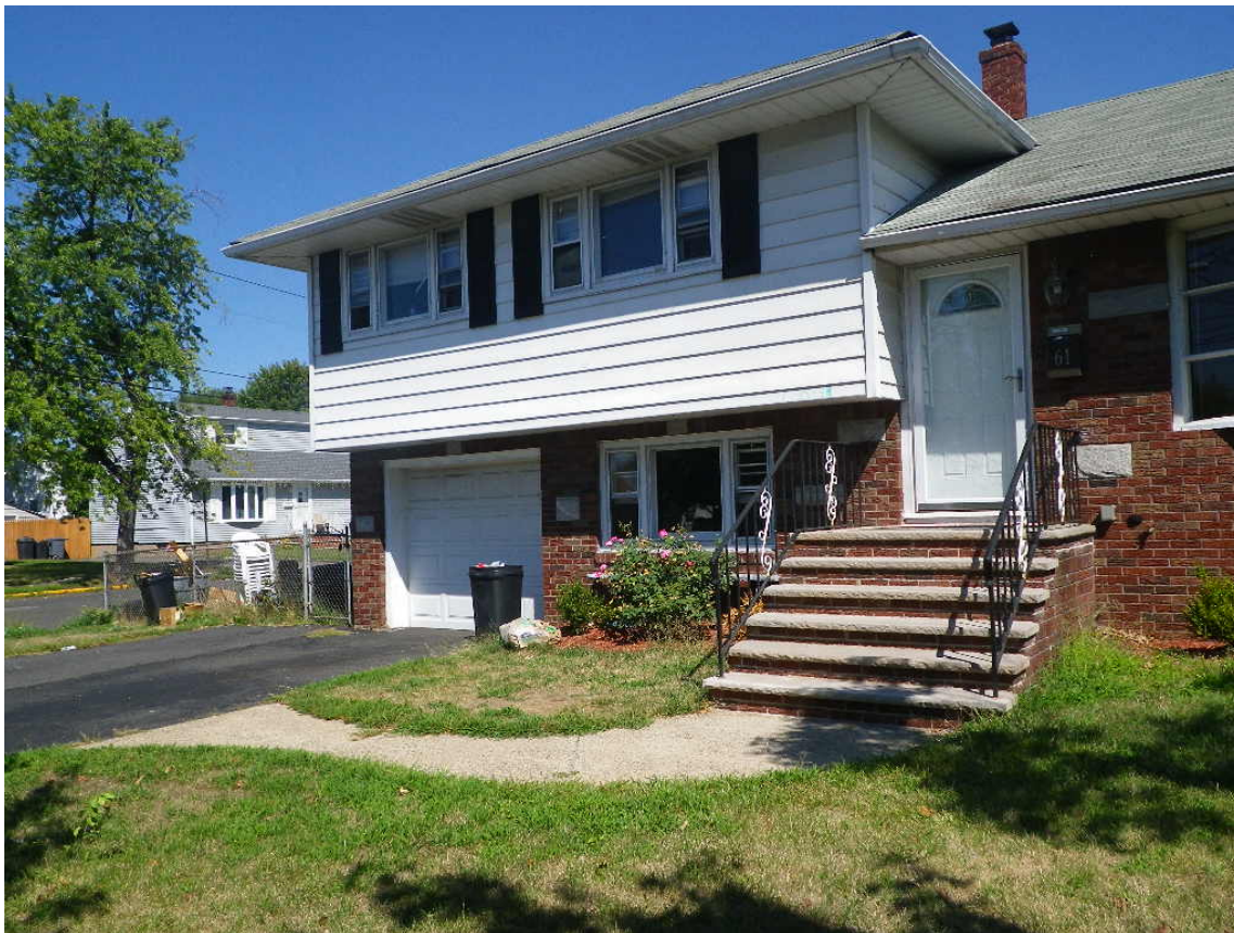
Fig. 2. 61 Trudy Drive, Lodi, NJ in September 2015. Hancock Street appears at the left of the photo, beyond the fence.
