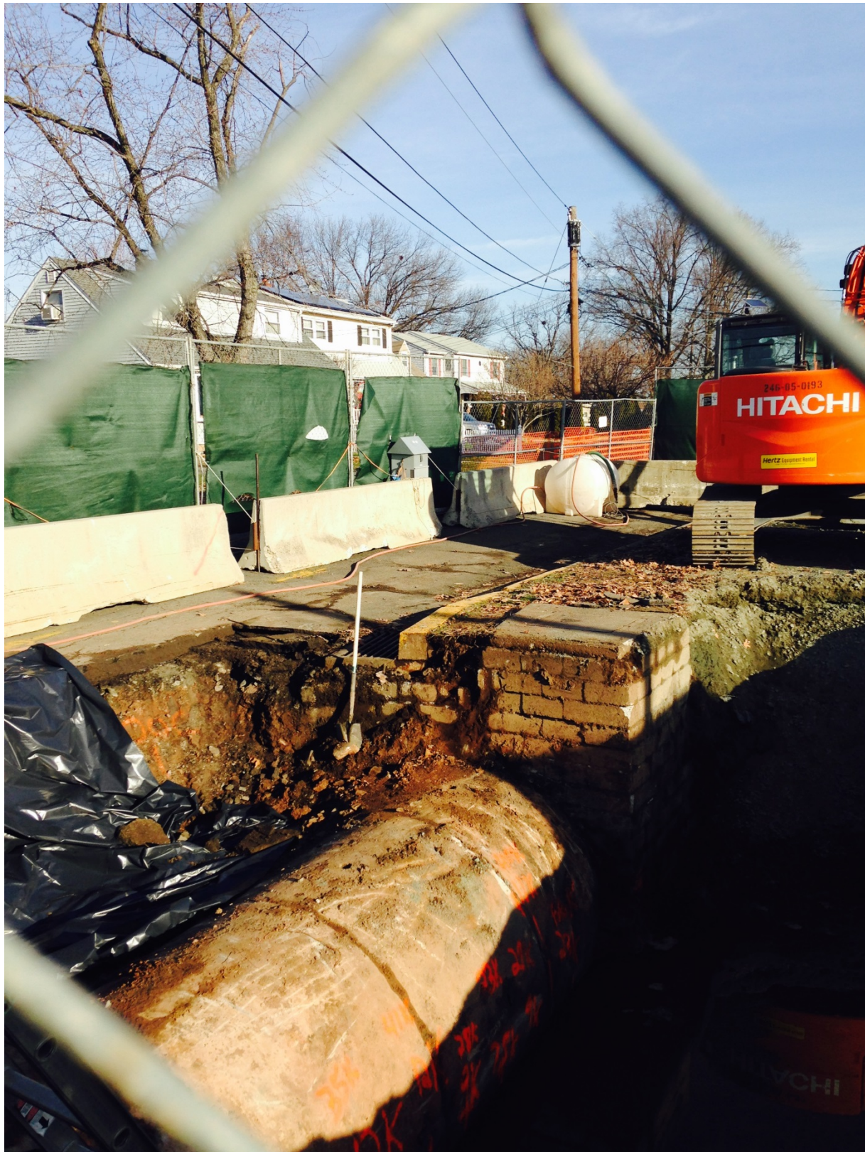
Figure 4. Soil around the Lodi Brook culvert pipe was also excavated during the 61 Trudy Drive remediation.
